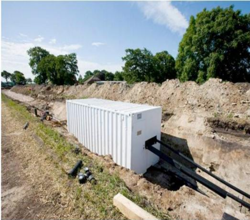
Figure 6.18: Typical Joint Bay Shelter
